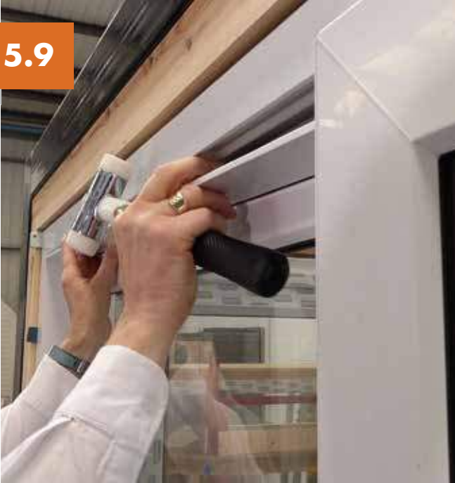
Head cover to be positioned last.
