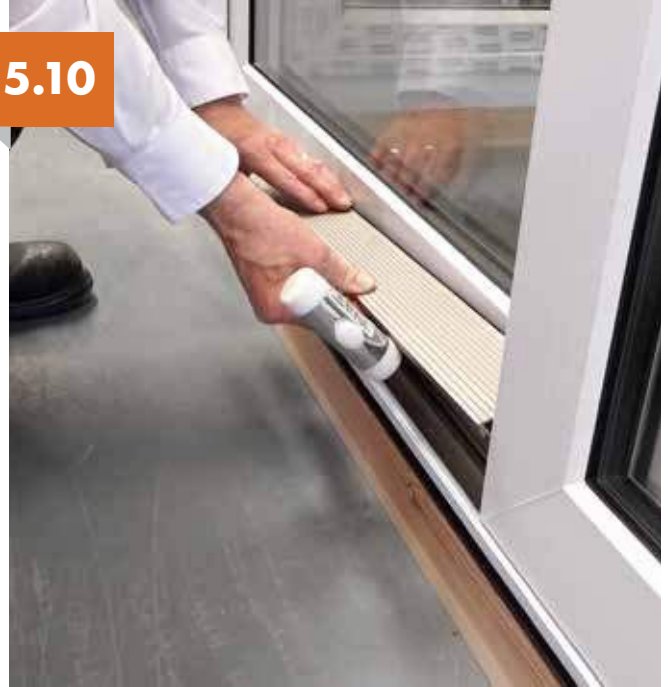
Position the cill cover/low threshold cover.
